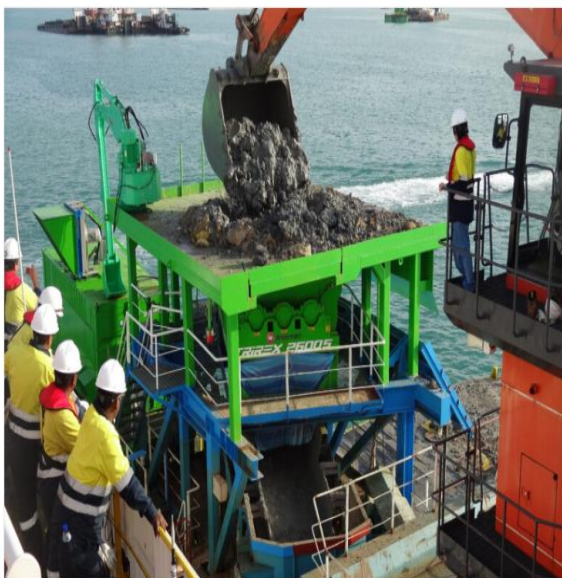
TRIREX 2600 S in dredging material
